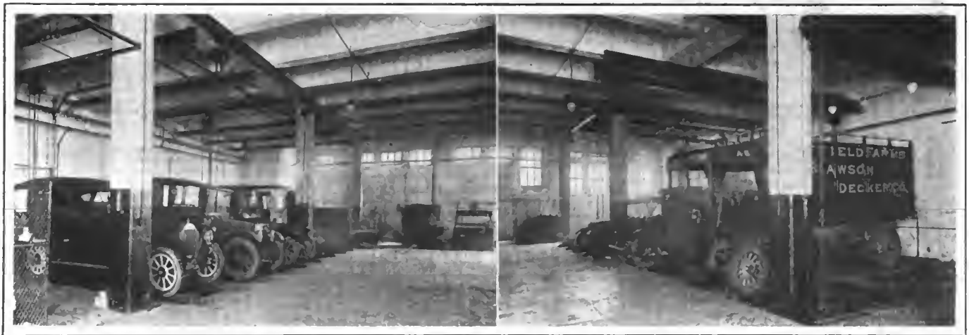
Panorama showing the interior of the first floor of the Perfection service building with passenger cars and trucks on the bays
